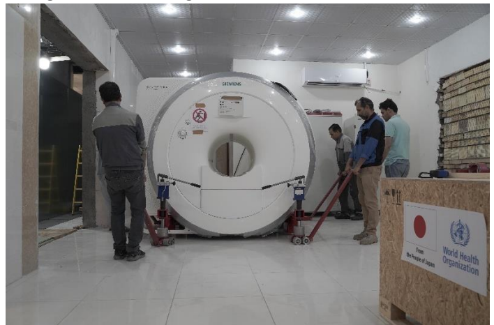
Fig. 8. Installation of MRI machine at Imam Ali hospital in Andimeshk, Khuzestan province. © WCO Iran
